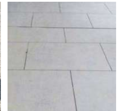
Concrete ashlar pavement to Mitchell Street
